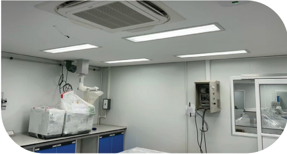
Installation of factory and building electrical systems.
