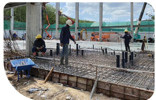
Structural and general construction work.
