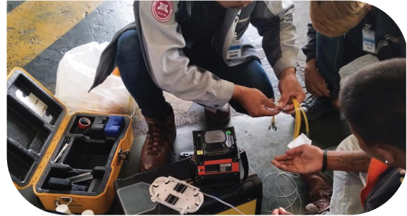
Installation of Wireless, WiFi, and PoE systems.
